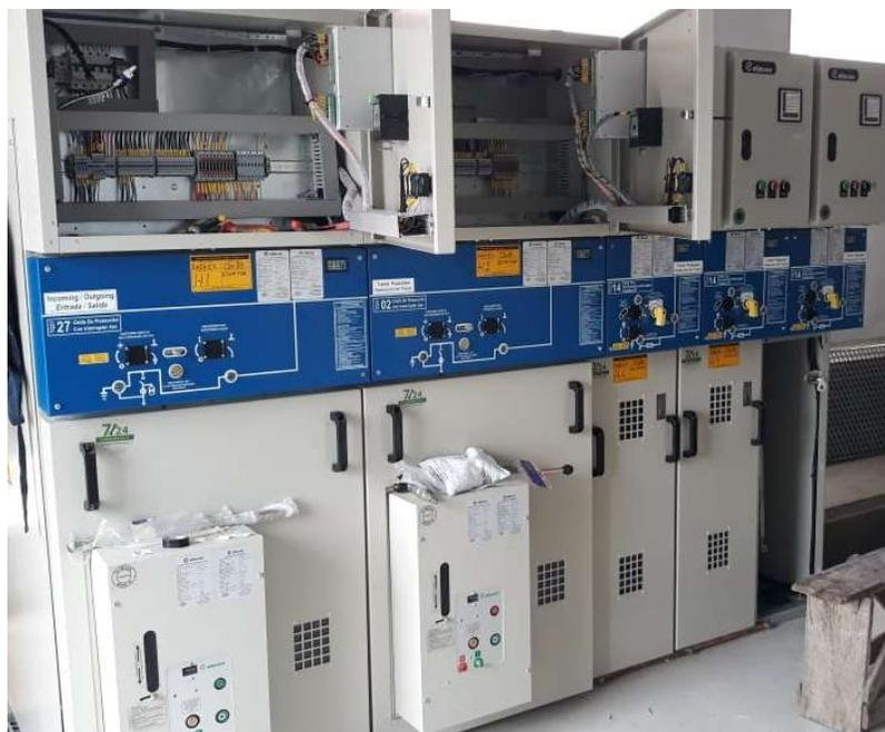
FIGURA 2.21 CELDAS DE MEDIA TENSION
