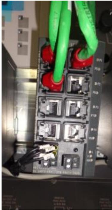
**Figura # 64 Switch scalance X208.**
