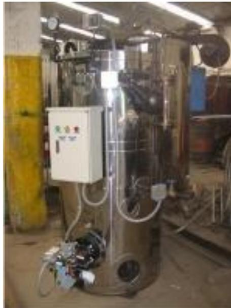
**Fig. 36 Caldera Piro-tubular Vertical 10 Bhp a Gas**
