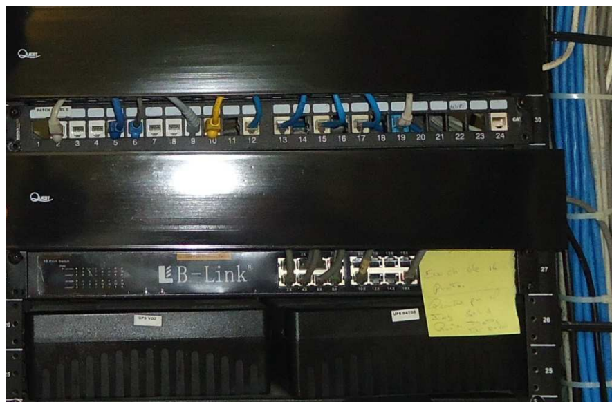
Figura 2. 23: Patch panel C y UPC's.
